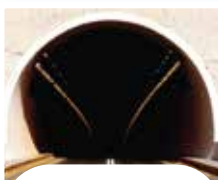
AIROLI-KATAI NAKA TUNNEL
