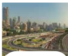
MUMBAI COASTAL ROAD MEGA PROJECT
